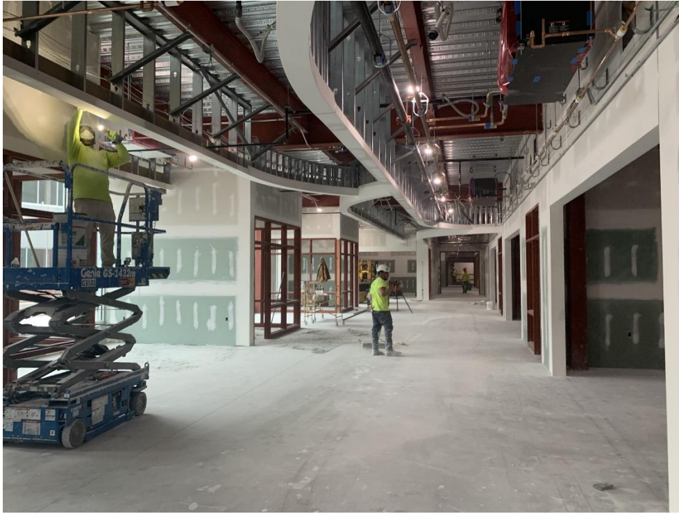
19. Area 4 – Gyp board install in first floor gradewalling neighborhood continues.
