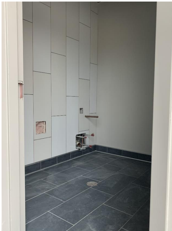
8. Area 6 – Floor and wall tile install continues.
