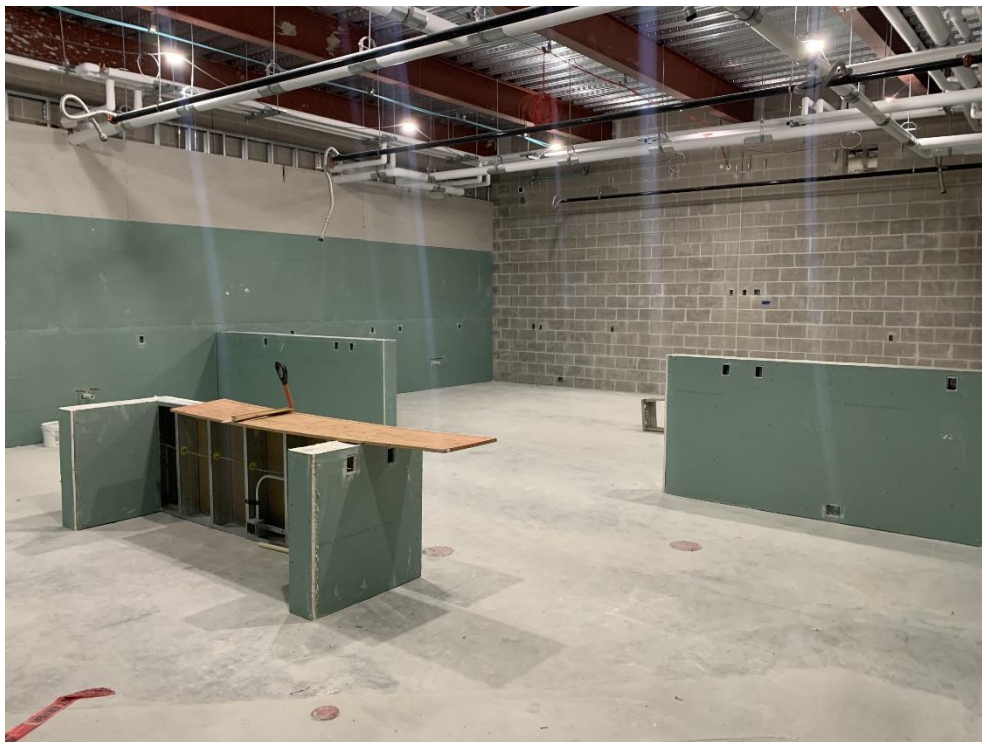
20. Area 3 – Gyp board install in culinary lab in progress.
